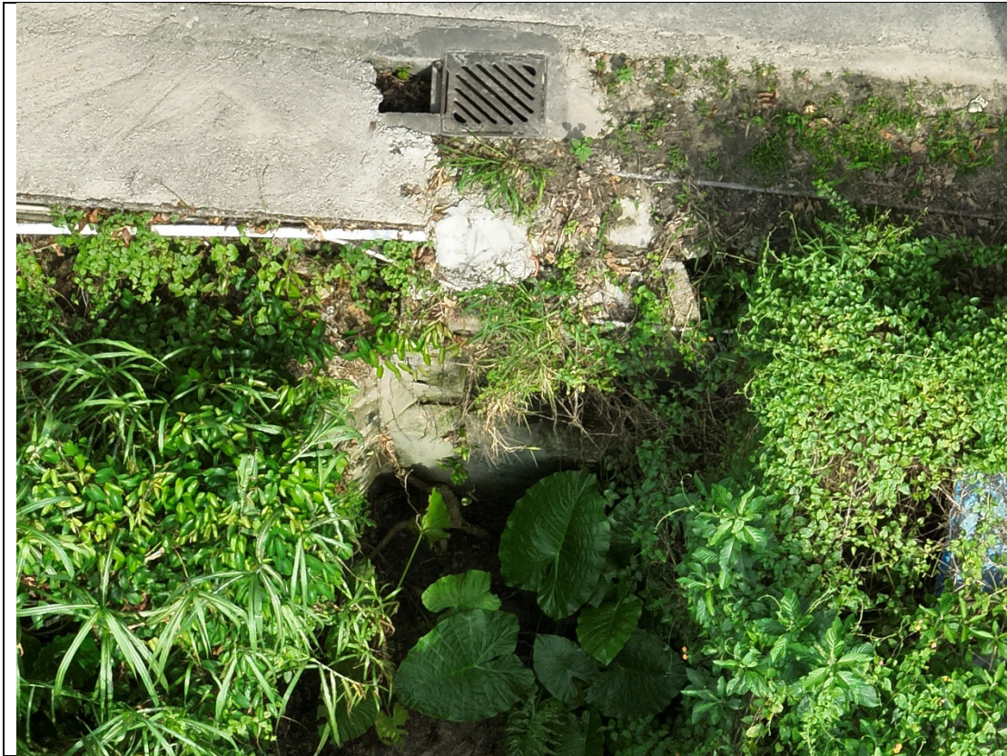
Photo 6 – Existing gully, manhole, 1200mm (approx.) underground pipe, and open drainage pit
